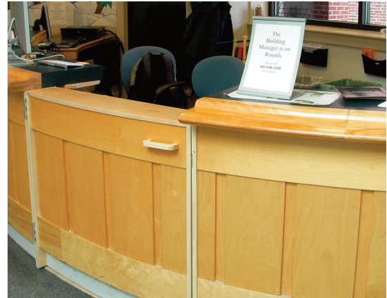
New door built into the Collis Info Desk.
